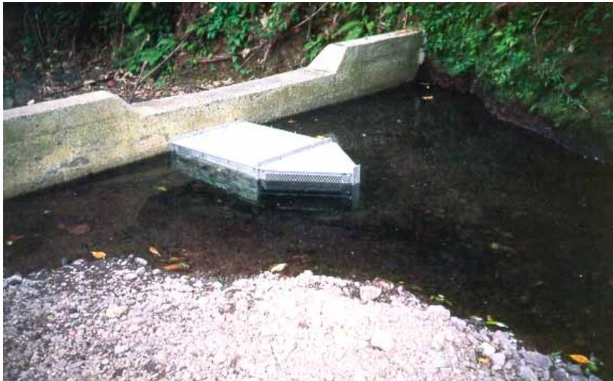
Concrete encased intake mouth to exclude leaves and debris
