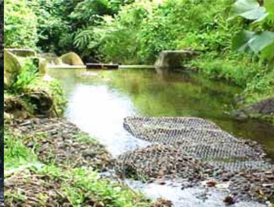
Wire mesh to cover the stones at intake
