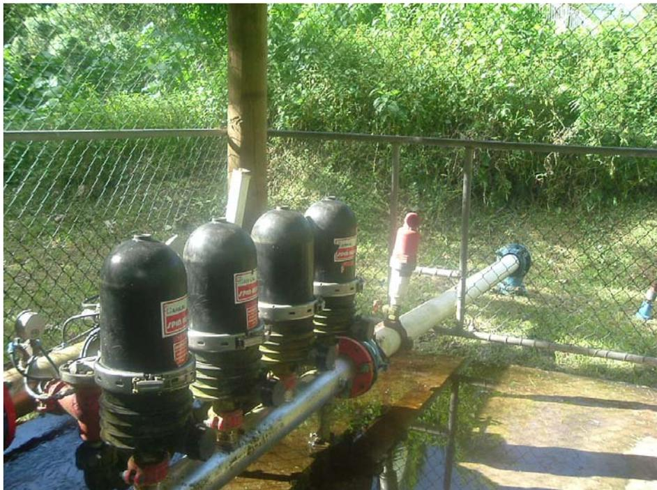
*20 micron ARKAL filters at Tupapa Intake*
