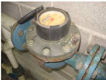
The value of bulk metering (and universal customer metering) cannot be underestimated. Without this basic but fundamental data on “how much” water and “where” it is flowing – it is near impossible to effectively manage a water supply system.
