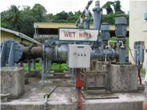
Photo: 3 Water from the two sources is collected at the Wet Well.
