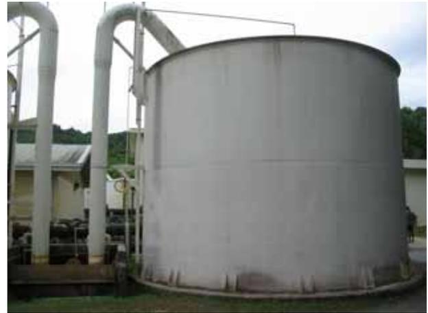
Photo: 4 Automatic Gravity Valve-less filters
