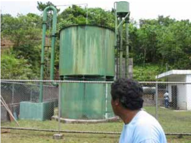
*Photo: 7 Treatment plant with an AGV filter in the foreground and the typical vegetation around the catchment in the background)*
