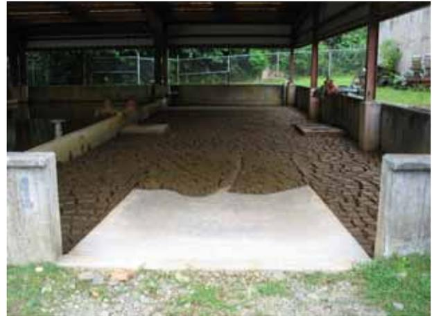
*Photo: 6 Sludge drying bed*
