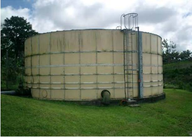
*Buffer tank (Steel bolted)*
