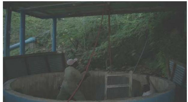
Two reservoir tanks are located on the hills close by the source which supplies water to the community and urban center through gravity mains. The storage tank capacities are 900 and 1100 cubic meter.
