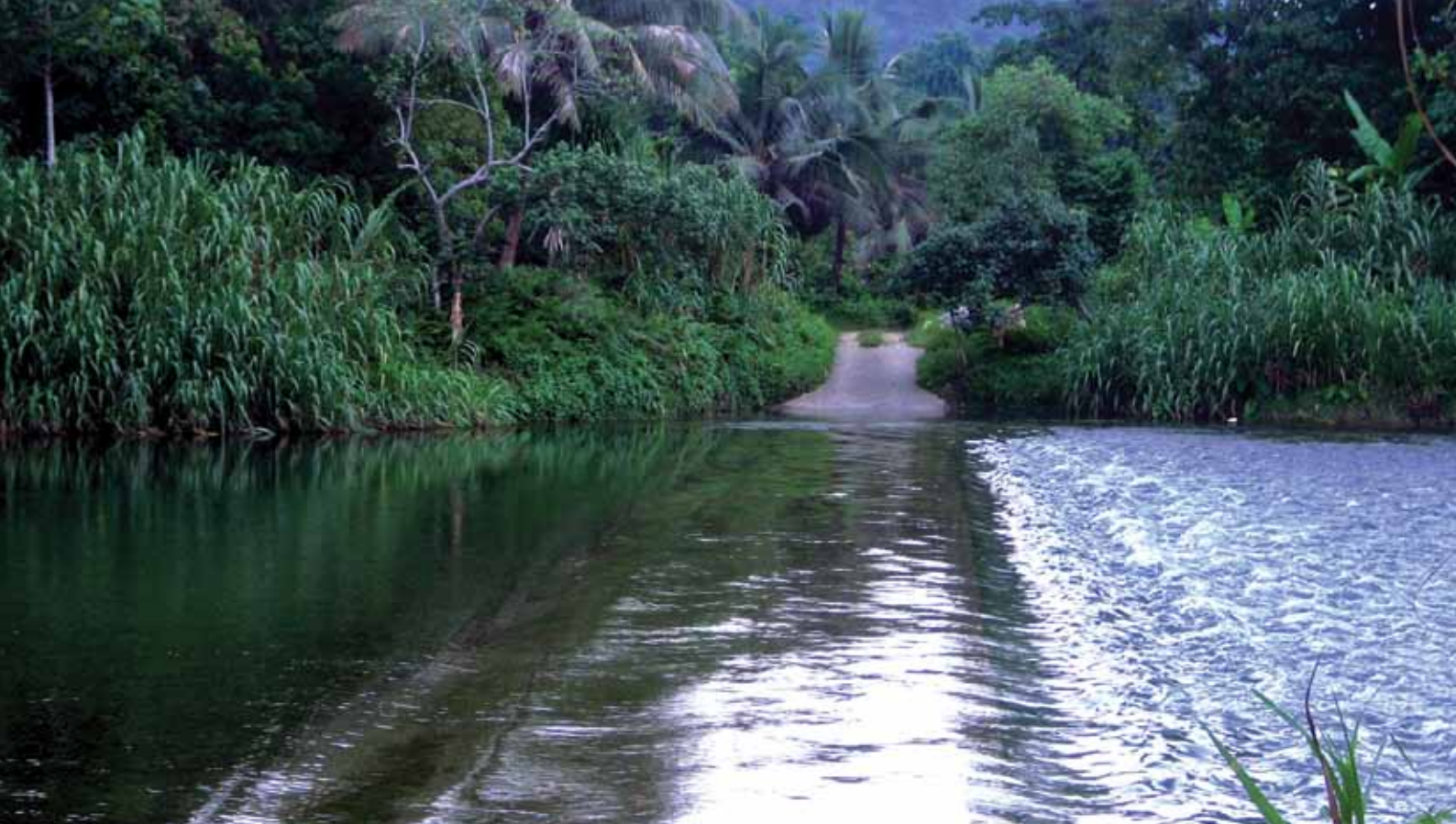
Lape River, Santos, road crossing
