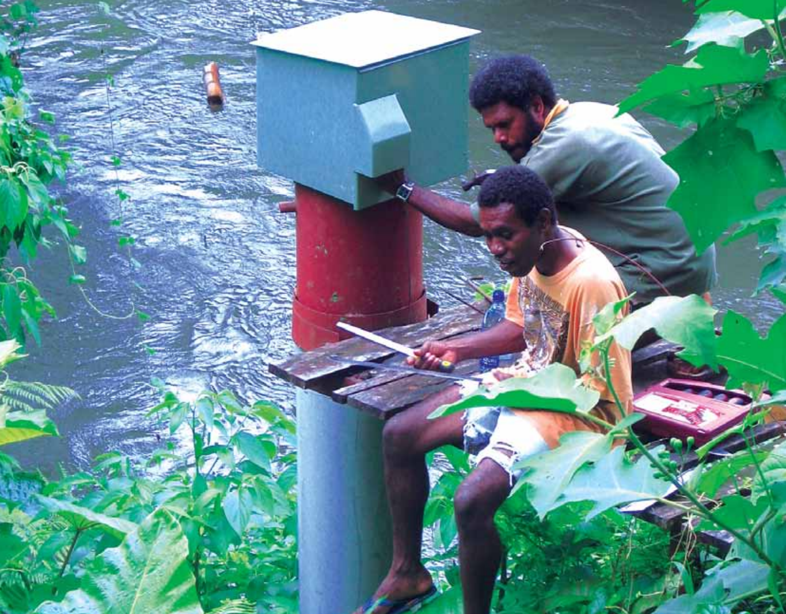
Sarakata river, Santos, station refurbishment
