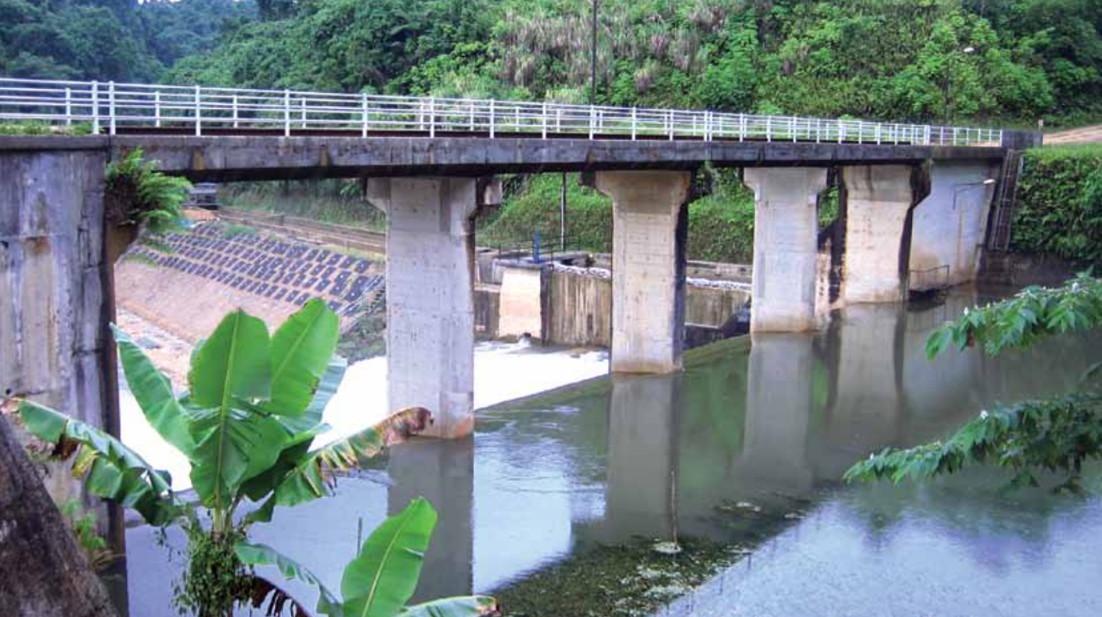
Sarakata, Hydroelectric power plant intake, Santos
