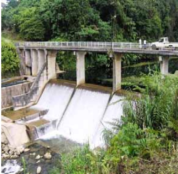
Sarakata River Hydro Dam
